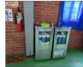
External photo(s) of the production unit(s) Water for workers.JPG
