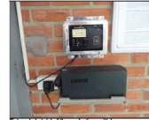
External photo(s) of the production unit(s) Fire record machine.JPG
